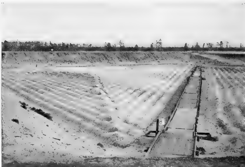
Fig. 45.—A sand filter bed ridged and furrowed for winter.
